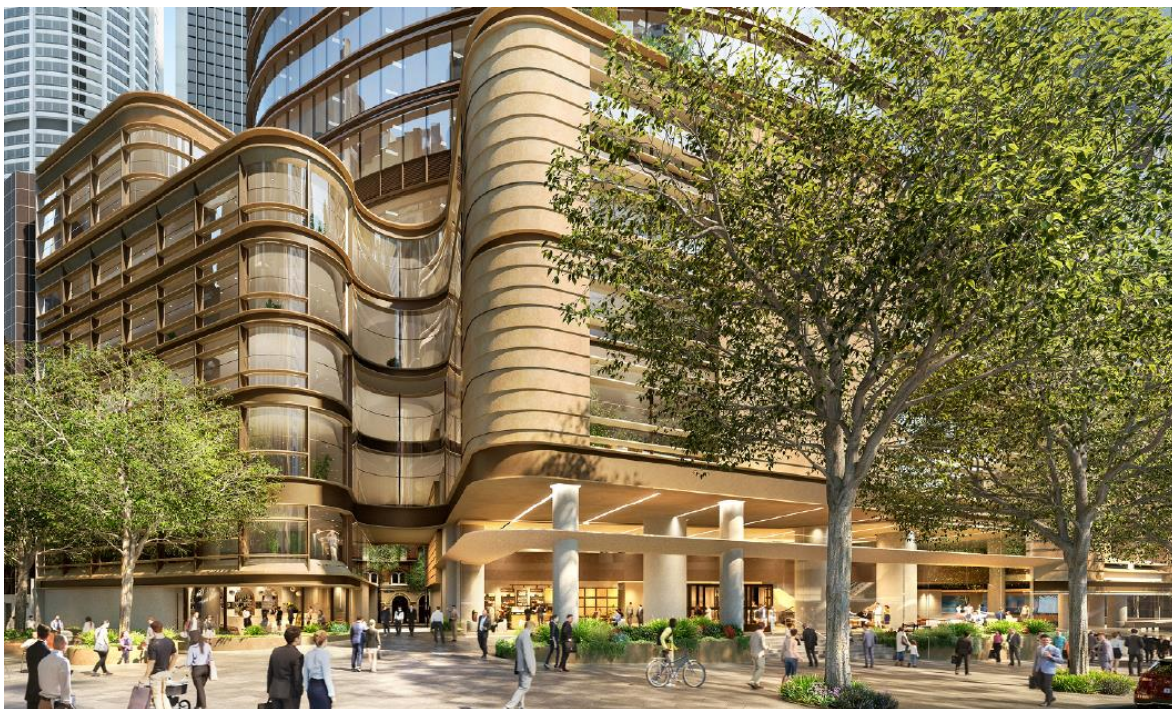
Figure 7: Indicative concept design of the through-site link looking through the future development towards Abercrombie Lane
